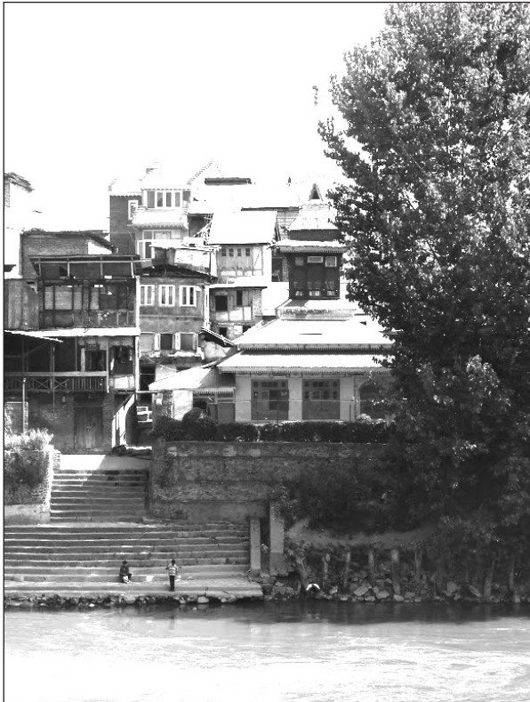
Fig. 10: Shrine of Shāh Ni‘matu ‘Allāh Qadri surrounded by a dense residential area, (© INTACH, 2010).
