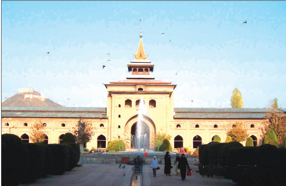
Fig. 9: Jāmi‘a masjid Srinagar, view across central courtyard, (© INTACH Kashmir, 2007).
