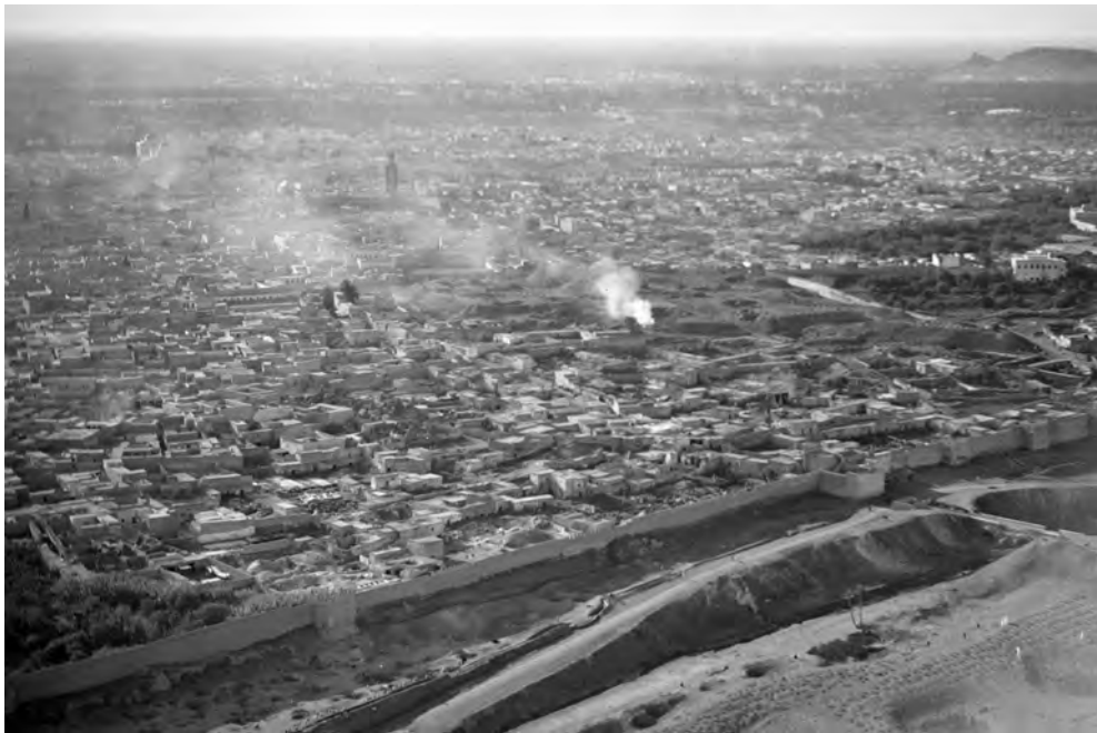
Fig. 2: Marrakech, aerial view of the tannery district, in the background the potteries and brickworks; city wall with bāb dbbāgh , kheṭṭaras , water channels and wād isīl with the old cemetery, 1930 (Photo: ETH-Bibliothek Zürich, Bildarchiv).
