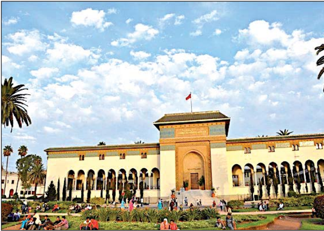
Fig. 2: Palais de Justice designed by Joseph Marrast for Casablanca's grand colonial plaza, 1925. The building consists of an open Moorish façade-arcade to an inner courtyard with an exquisite play of local archaeological details following a classical subdivision centred around a monumental Roman-arched gate (Photo: Author, 2009).
