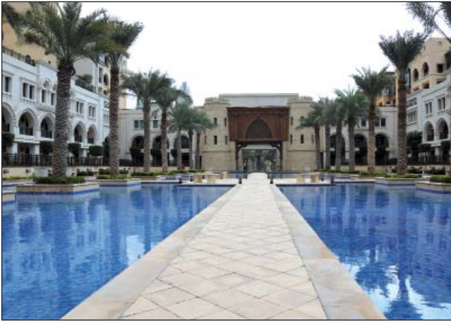
Fig. 12: The main entrance of Old Town Island and its Palace Hotel in Dubai. The town was designed and implemented by Emaar (2007). The Town presents an amalgam of eclectic Arabic and Islamic idioms to fabric an image of a madina. The design is extravagant and without consideration of the authentic different traditional styles (Photo: Author, 2010).
